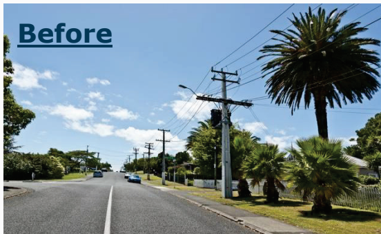
Udys Road before the undergrounding and power pole removal.
